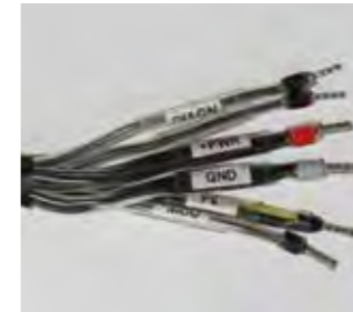
Cable termination The power/signal cable wires are crimped at the free flying end.
