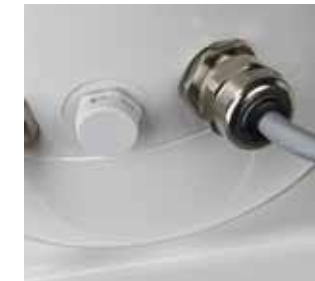
Cable entry cable entry for the supply cable is from the side of one of the light units.
